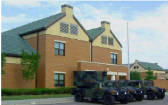
Fort Bragg Airforce Base, USA (Exhaust)
